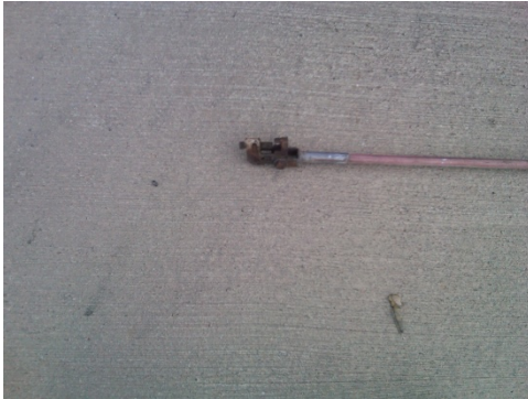
Broken Unipole Skirt Bracket
